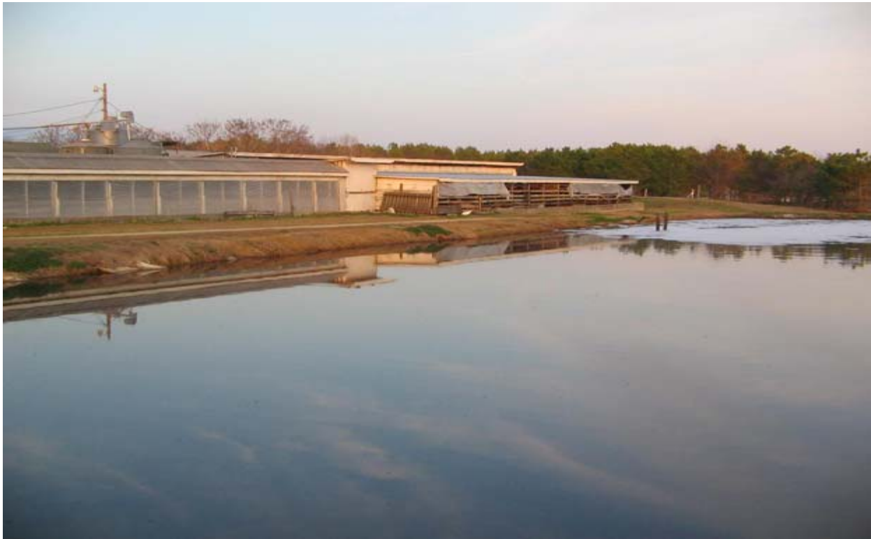
Figure 3: Appearance of the hog lagoon after 60 days of the trial. Note that no sludge is breaking the surface and that all shoreline sludge and foam are no longer present.
