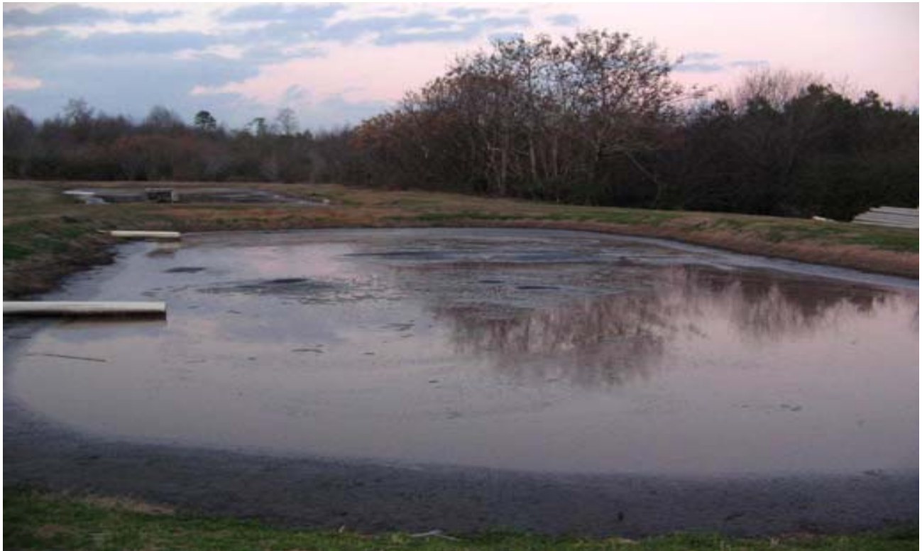
Figure 1 – Small hog lagoon in North Carolina. Sludge in the lagoon reached all the way to the surface of the lagoon when we arrived.
